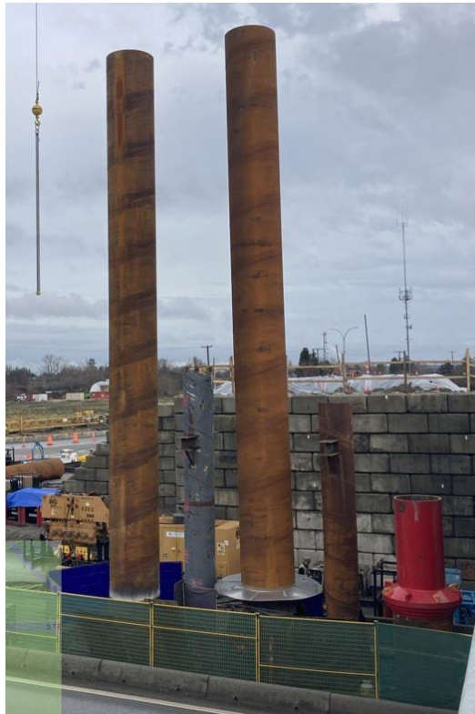
Figure 1 Pier Pile Welding at Northeast Quadrant
