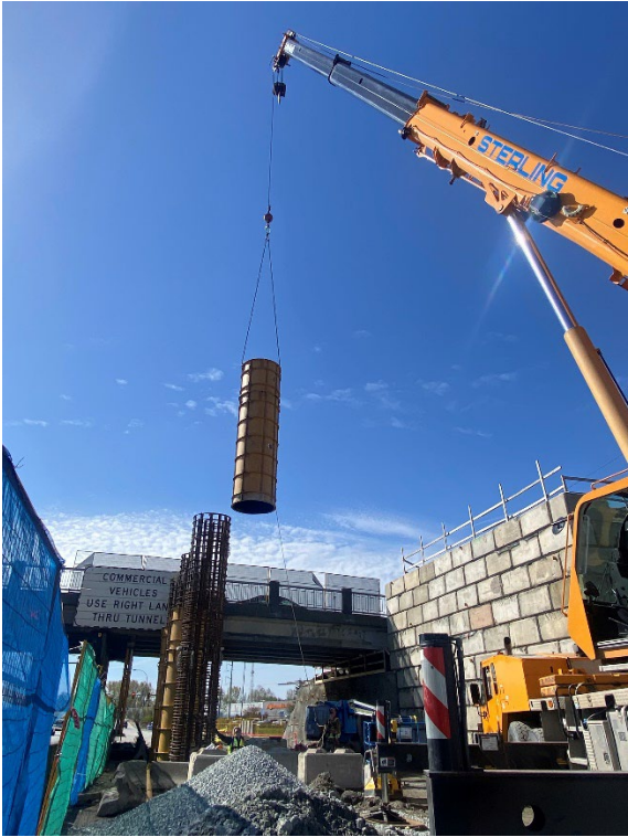
Image 1: Lifting pier column formwork – NW quadrant
