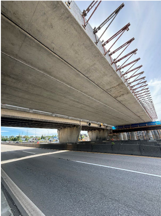
Image 2: Main-span girders over Highway 99, facing west
