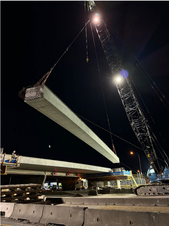
Image 1: Heavy-lift crane hoisting one of the 50-tonne girders into place
