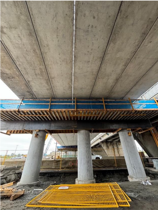
Image 1: Newly installed end-span girders on the northwest side.
