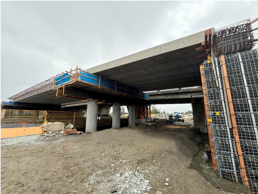
Image 3: New end-span girders installed between the northwest abutment and main-span girders.
