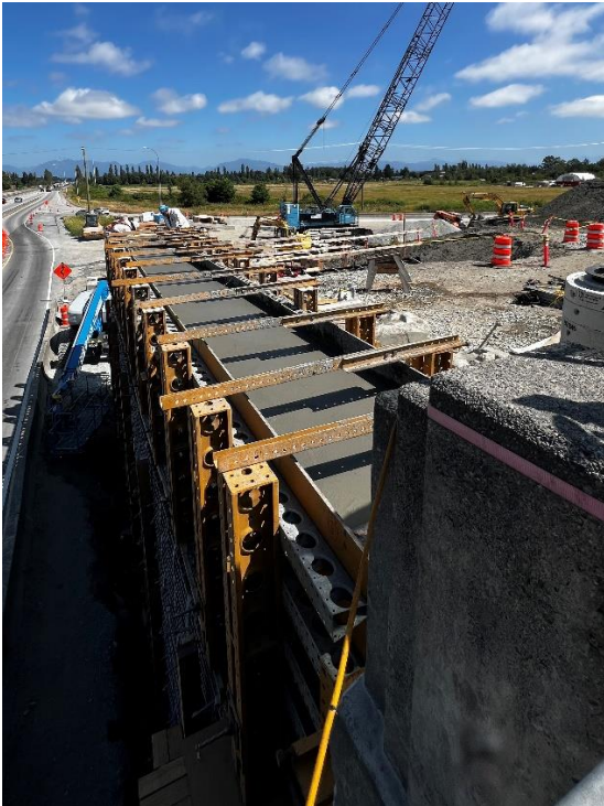
Image 2: Preparing northeast abutment cap for end-span girder installation.
