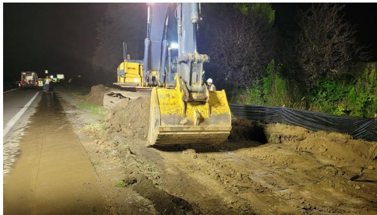
Preloading of soil along Highway 99 in Richmond (September 6, 2024).
