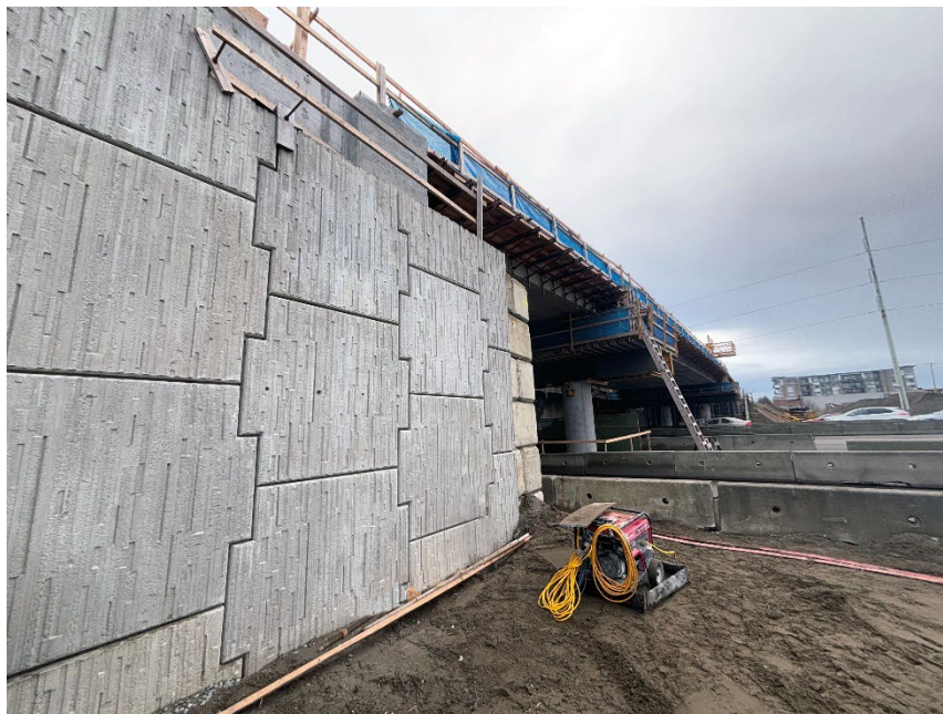
Figure 3: Concrete panels on the Phase 1 east approach.
