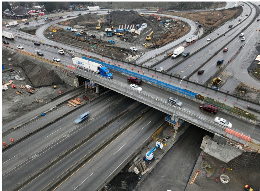
Figure 3: East and westbound traffic on the new Phase 1 structure facing south.
